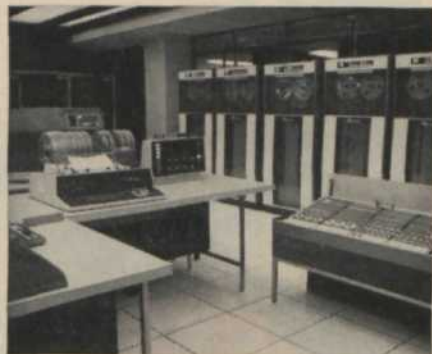
This is the insurance company's modern data processing installation.
